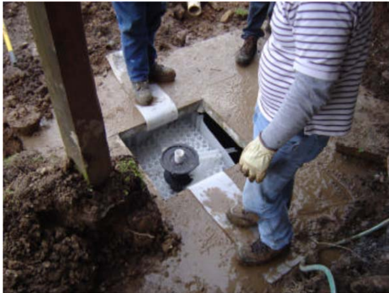
Figure 3.4: RetroFAST unit installation in an existing septic system
