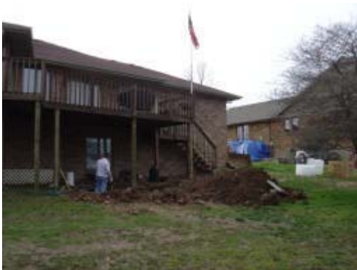
Existing tank uncovered
