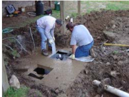
RetroFAST lowered in the tank.
