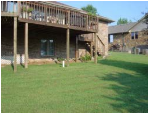
Septic tank and chamber lateral field
