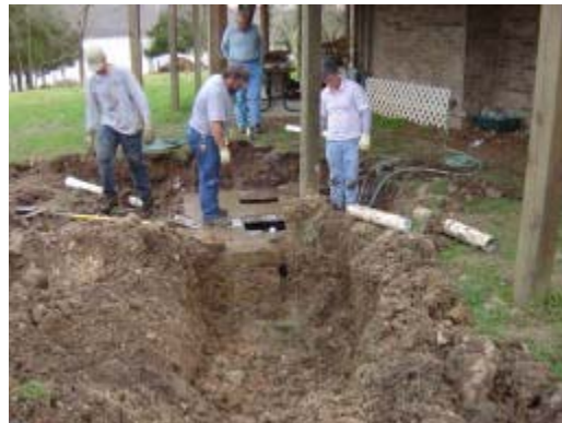
Square access hole cut in tank lid
